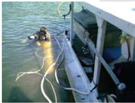
Diver is setting an airbag to raise the vessel.
